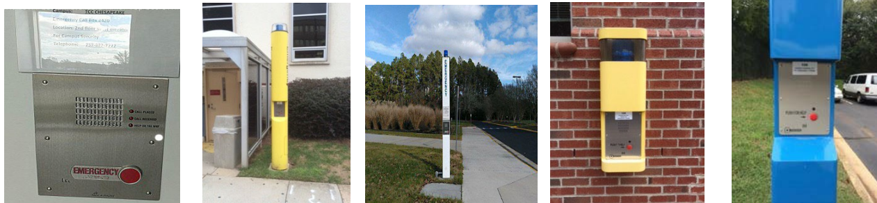
Figure 1. Emergency Call Boxes
